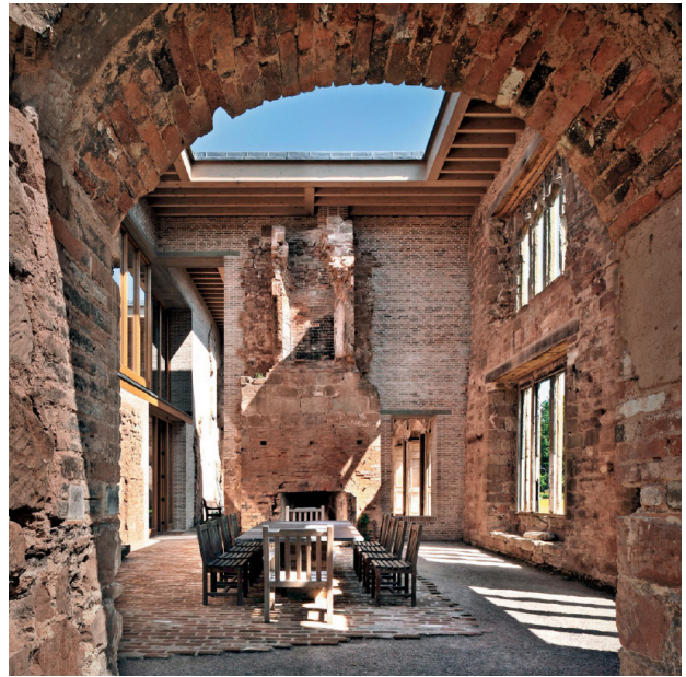
Fig. IV-01. Umbau Astley Castle da Witherford Watson Mann @DETAIL
